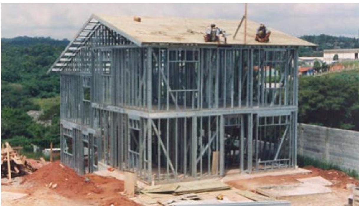
**Figura 4:** Light Steel Frame (LSF)
